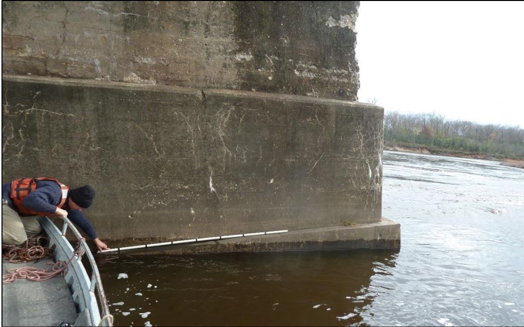
Figure 2: measuring pier rotation
