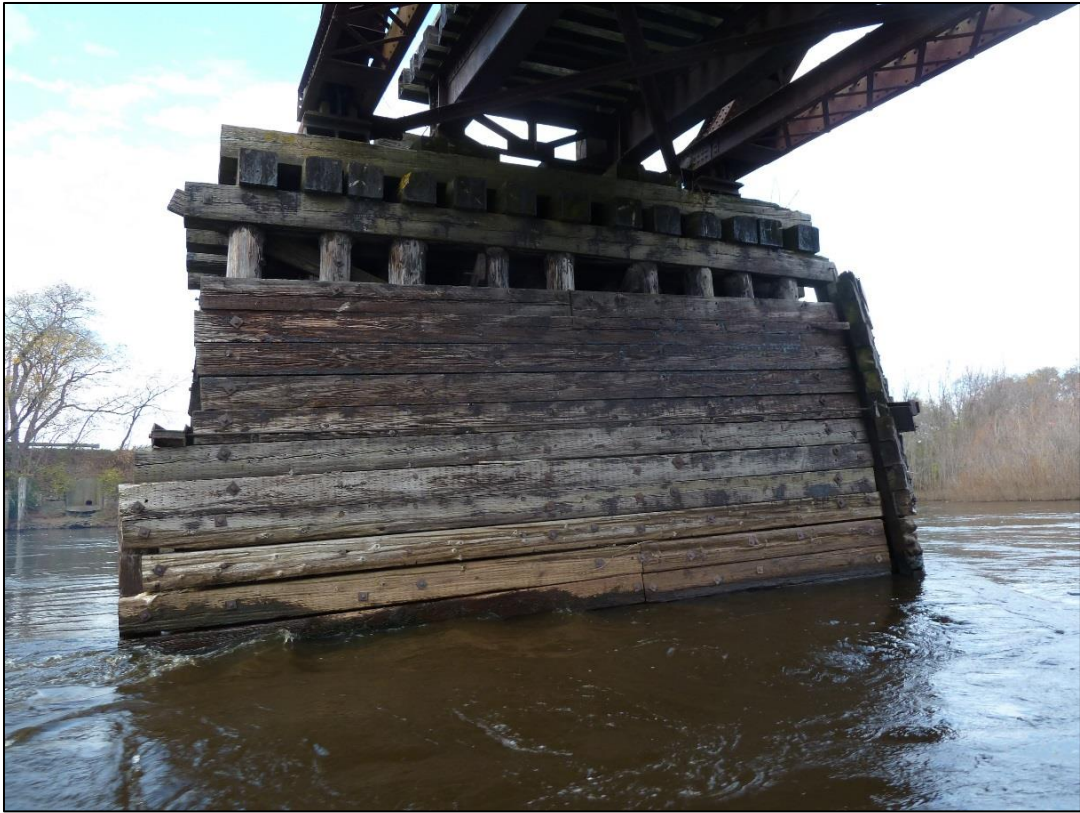
Photo 15: Pier 3, east face
