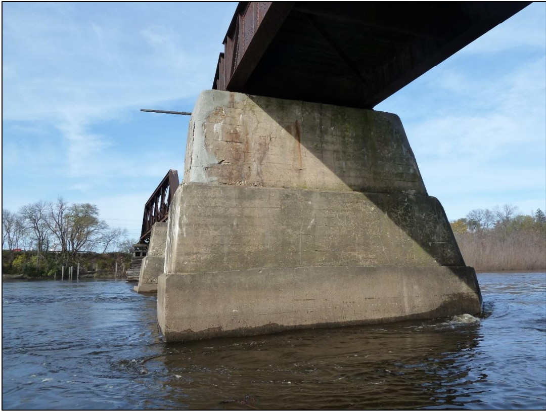
Photo 7: Pier 1, east face
