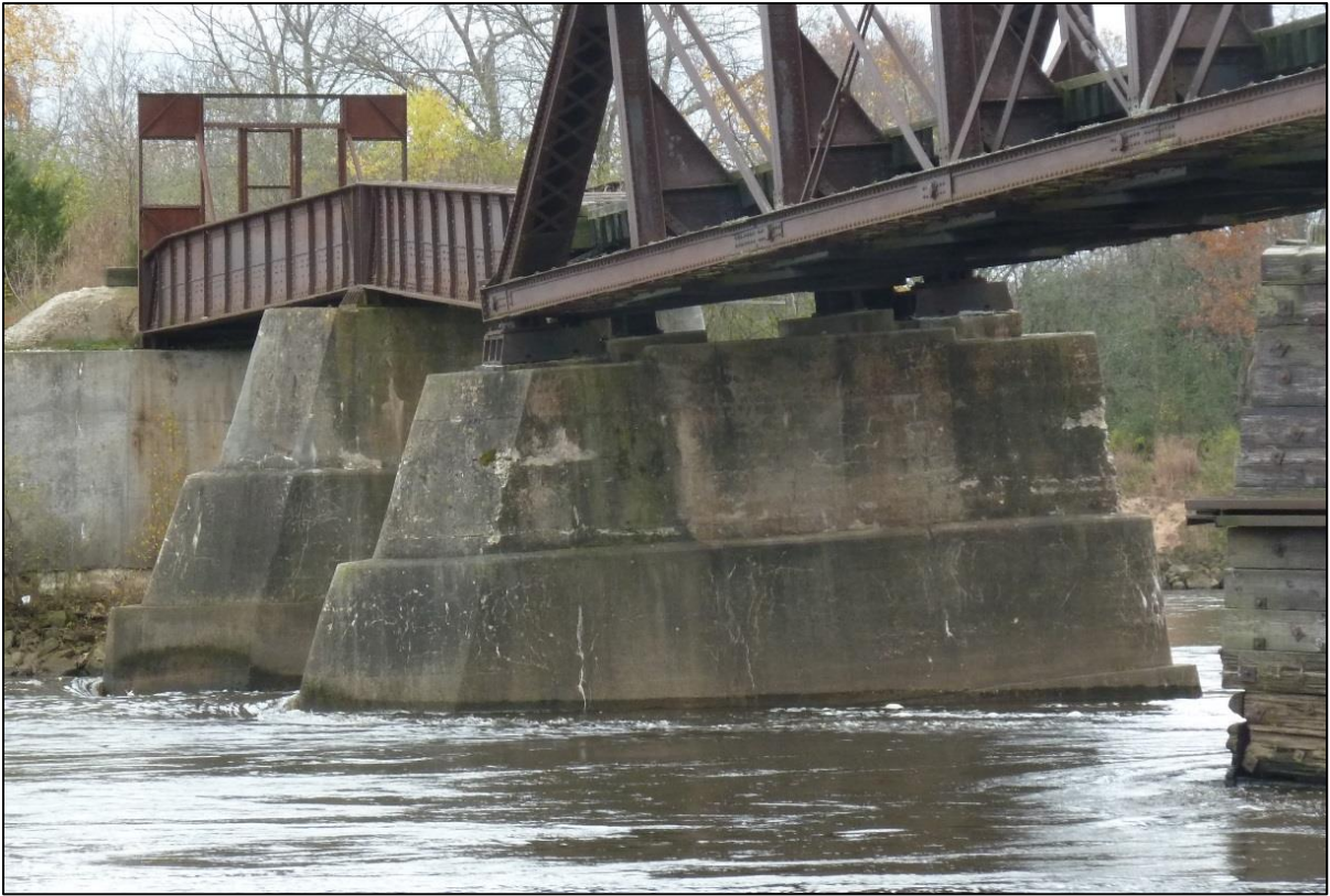
Photo 11: Pier 2, west face
