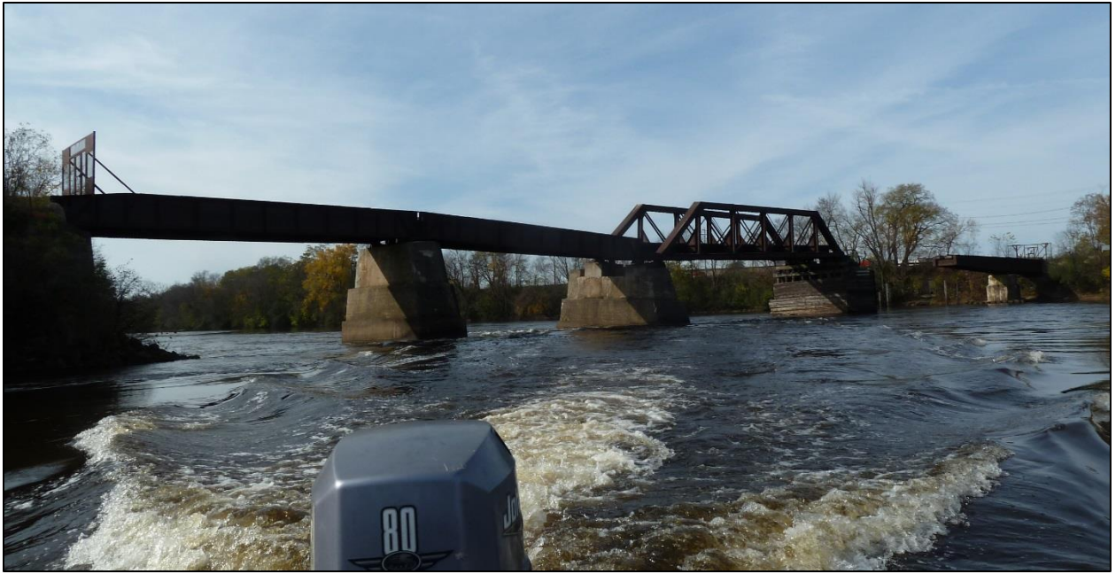
Photo 1: upstream elevation—view from east side
