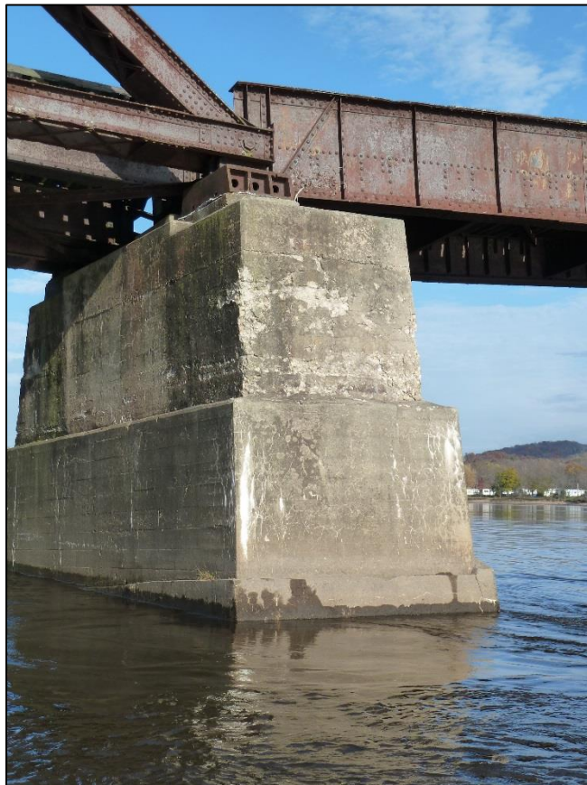
Photo 10: Pier 2, downstream face
