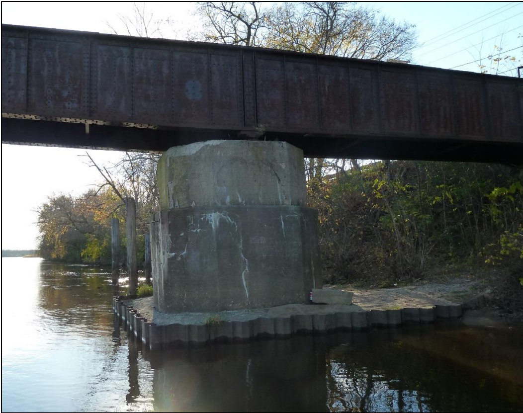
Photo 17: Pier 5, upstream face
