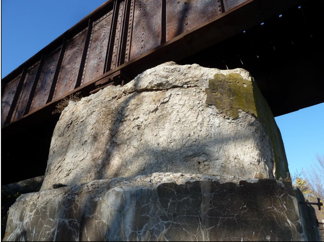
Figure 7: Pier 5 shaft, downstream face
