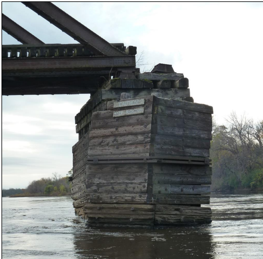
Photo 16: Pier 3, upstream nose
