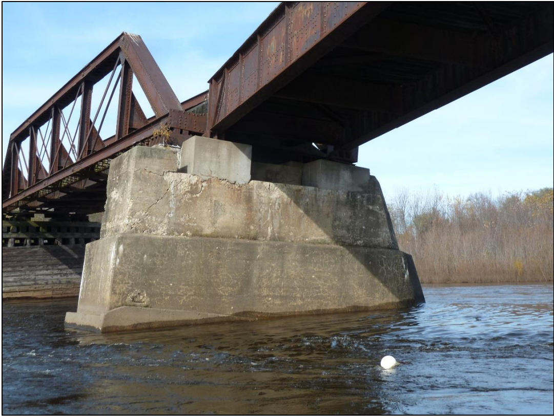
Photo 9: Pier 2, east face
