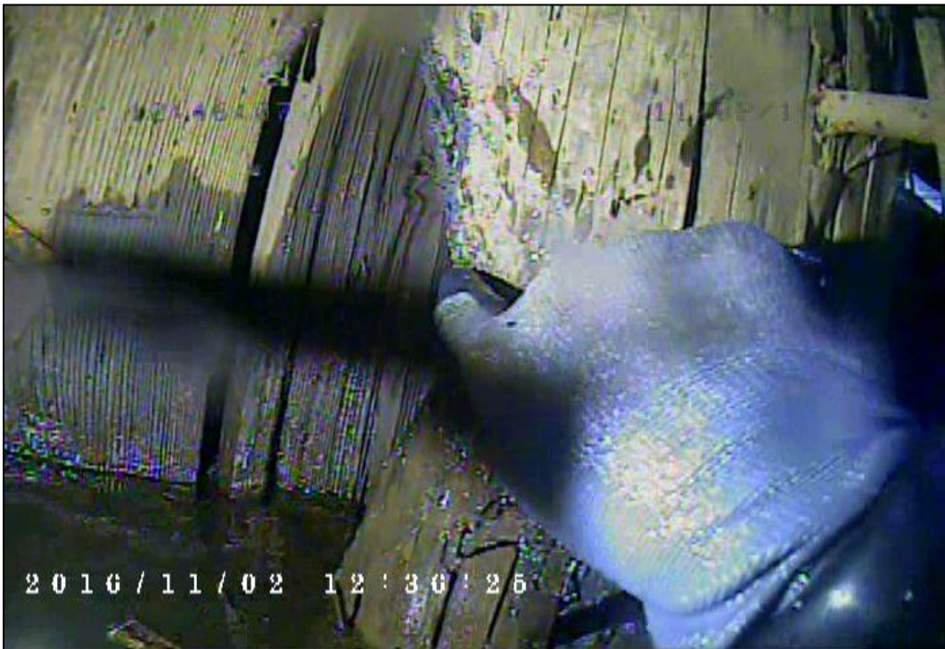
Figure 5: abraded pile, east side of pier
