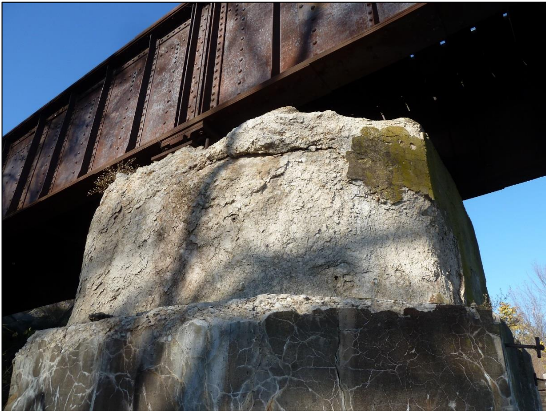
Photo 18: Pier 5, downstream face
