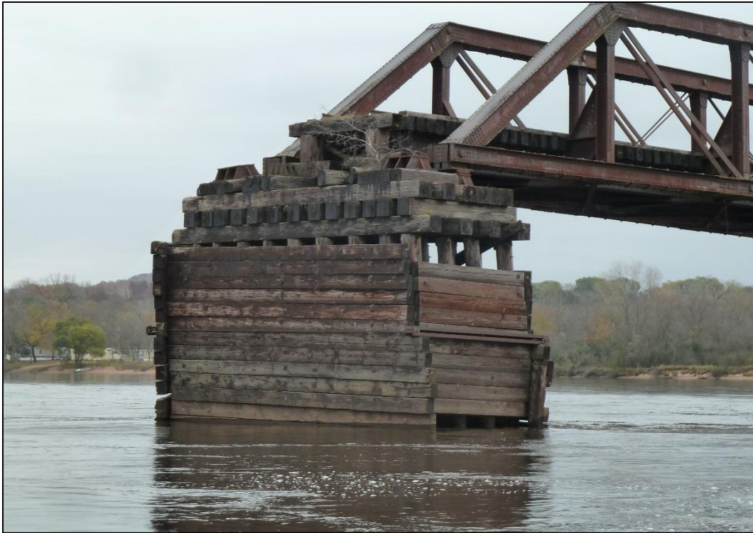
Photo 13: Pier 3, west face
