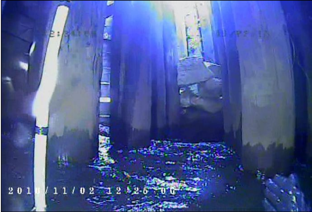
Figure 4: riprap placed inside pier at nose
