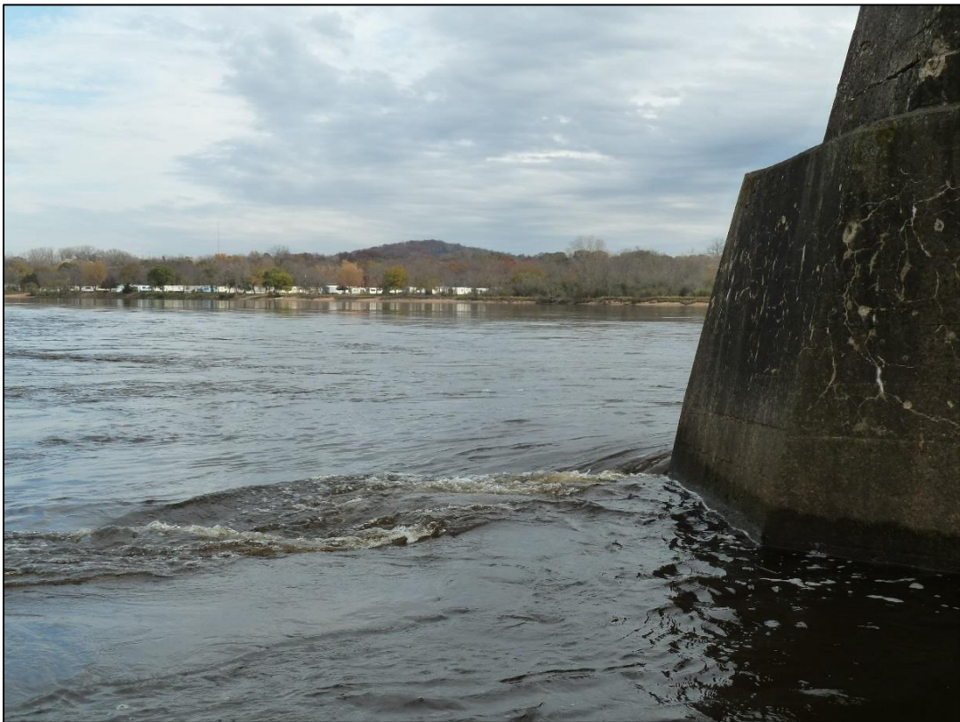
Photo 12: Pier 2, eddy formed west side of nose
