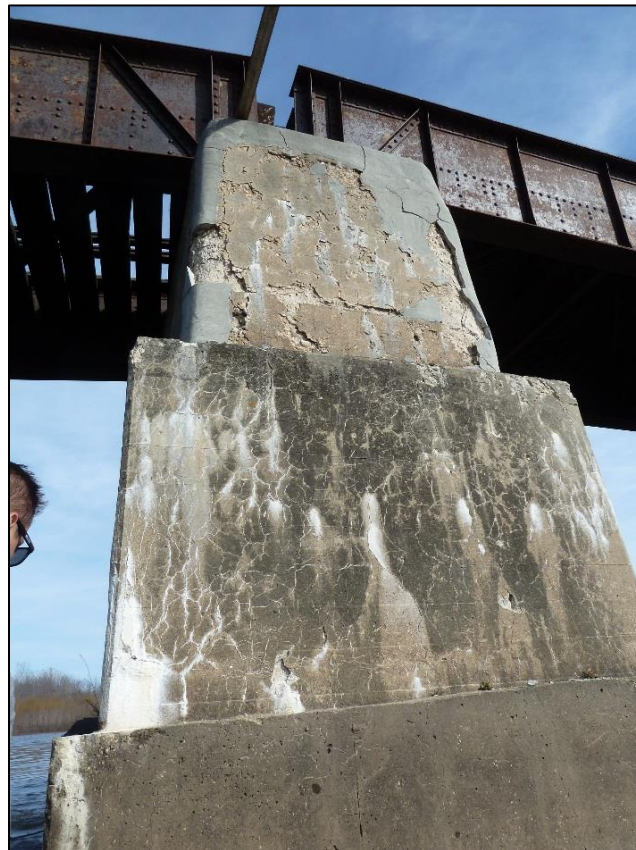
Photo 8: Pier 1, downstream face
