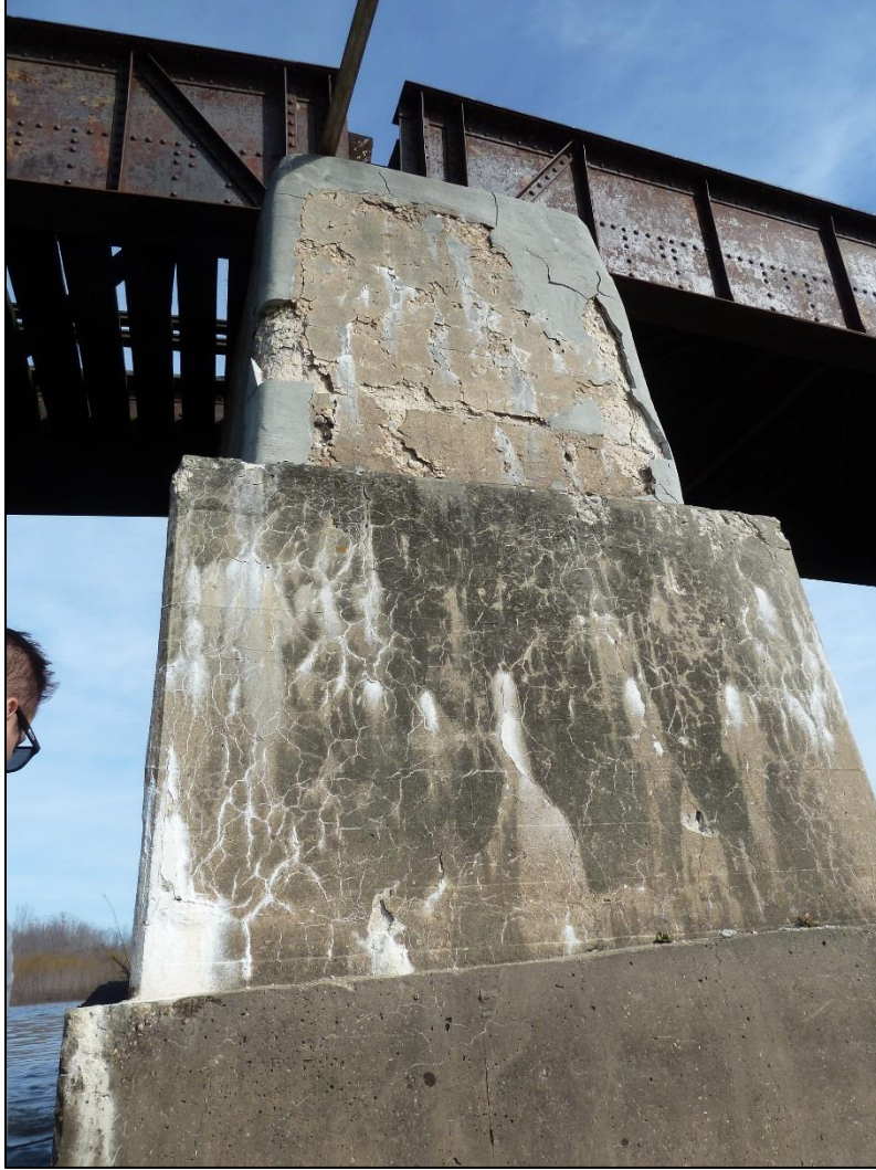
Figure 1: Pier 1 shaft, downstream face
