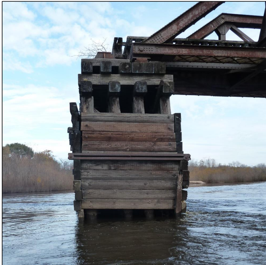
Photo 14: Pier 3, downstream face
