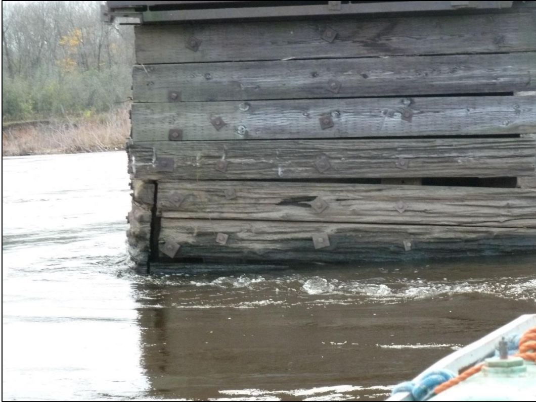
Figure 6: condition of perimeter timbers at nose
